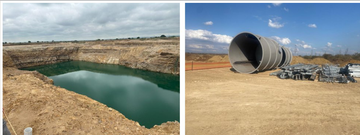
Fig 2: Development on site
